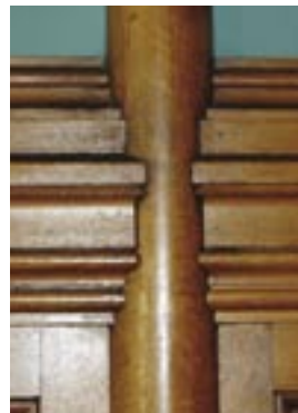
In downtown St. Paul, the Landmark Center (home of the AAW offices and gallery) has many examples of fine turning. These 9-foot oak columns have a slender taper and curve and fascinating scribing detail with wall panels.
